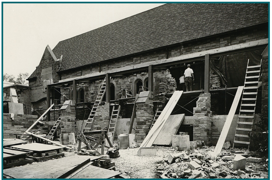
1960's Sanctuary Widening Project. The original walls were once where today's arches stand. The balcony was also added.
